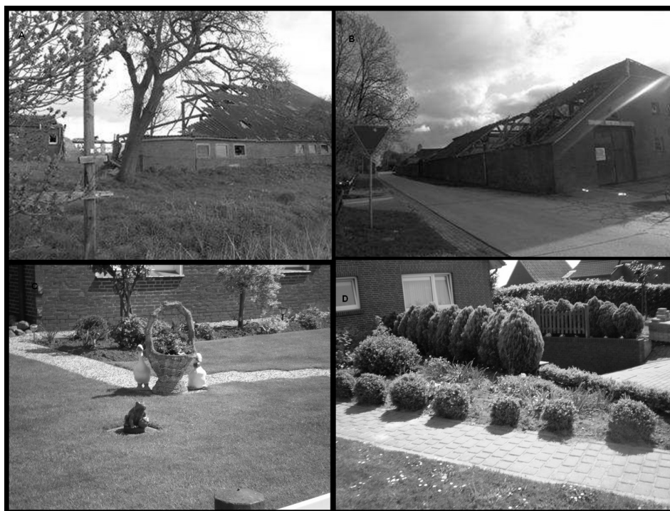
Fig. 2. A., B. Devastated buildings and facilities in an abandoned agricultural farm. C,D. Standardised stylisation of traditional rural gardens, being a result of ignorance towards the tradition of the place. The Diztumhamrich settlement, East Frisia.
