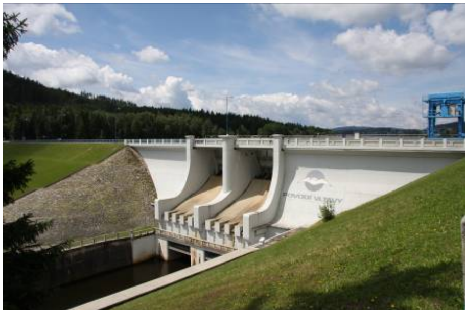
Phot. 5. Dam from the bottom water (photo by R. Kujawa)
