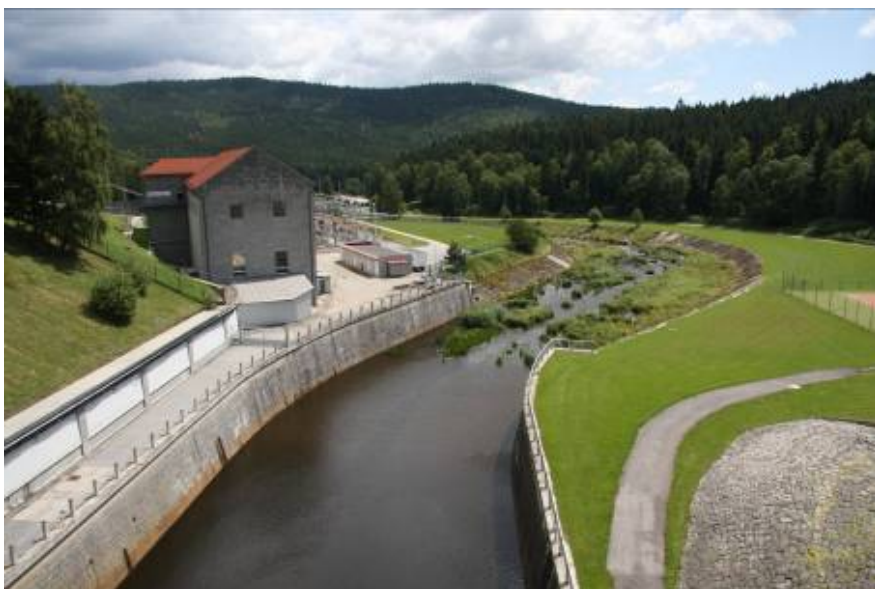
Phot. 6. Strengthened river bed below the dam (photo by R. Kujawa)
