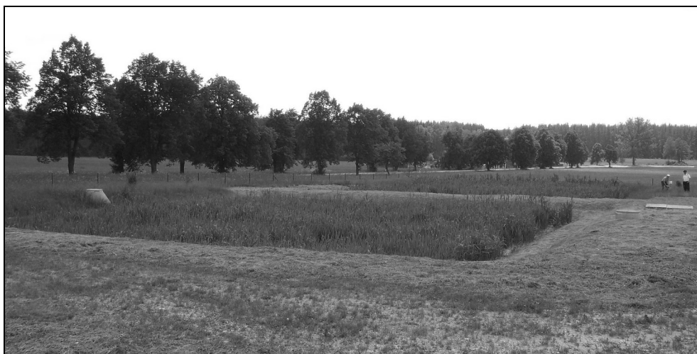
Phot. 2. Vertical flow constructed wetland (phot. Dąbrowski 2010)
