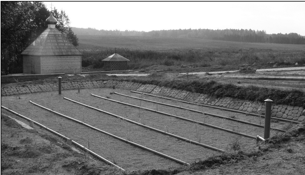
Phot. 1. Vertical flow constructed wetland (phot. Ekoprom 2011)
