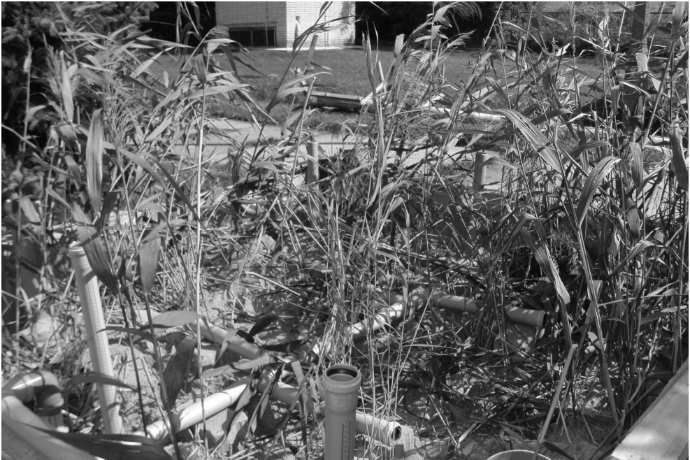
Phot. 5. Constructed wetland after planting (phot. Tomczuk 2010)
