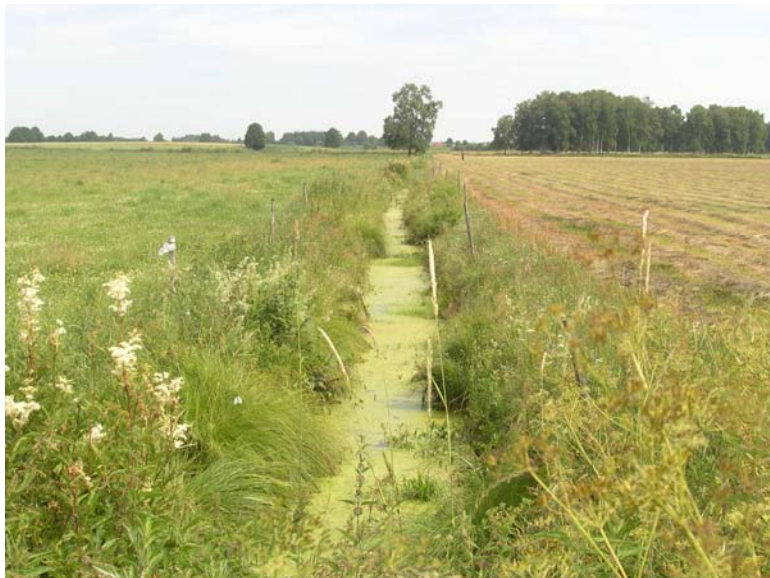
Phot. 2. Non-conserved melioration ditch does not act drainage-irrigation functions on the object © A. Kiryluk
