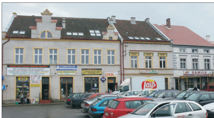
Fig. 2. A compact row of houses along one side of the main market square Source: the authors
