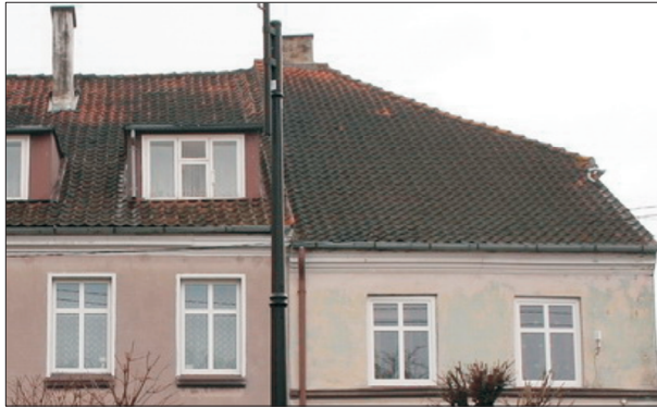
Fig. 9. A mansard roof
