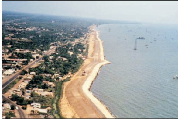
Fig. 1. Protective earth dyke
