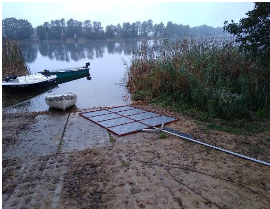
Photo 8. Stabilizing plate of the outflow pipeline.
