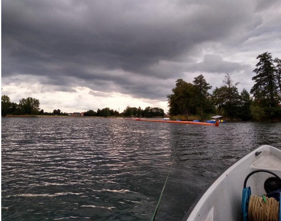
Photo 9. Outflow pipeline during installation.
