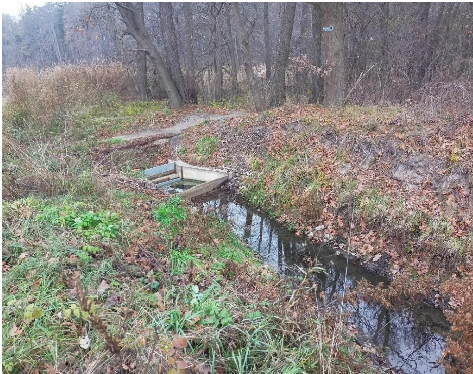
Photo 11. Northern dam (Inlet).
