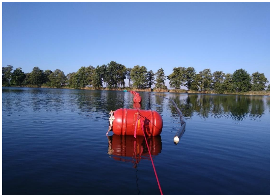
Photo 5. Installation of the underwater curtain.
