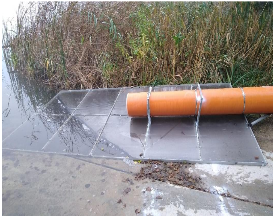
Photo 6. Filling pipeline and its inlet drop plate.
