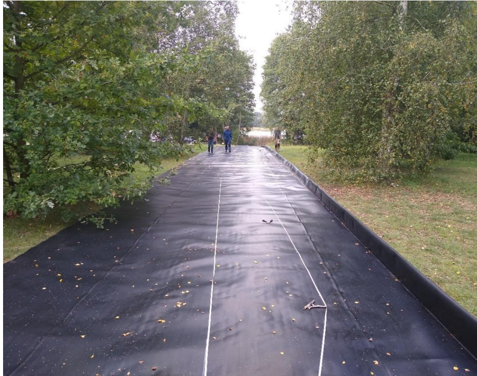
Photo 4. The installed HDPE geomembrane (curtain).
