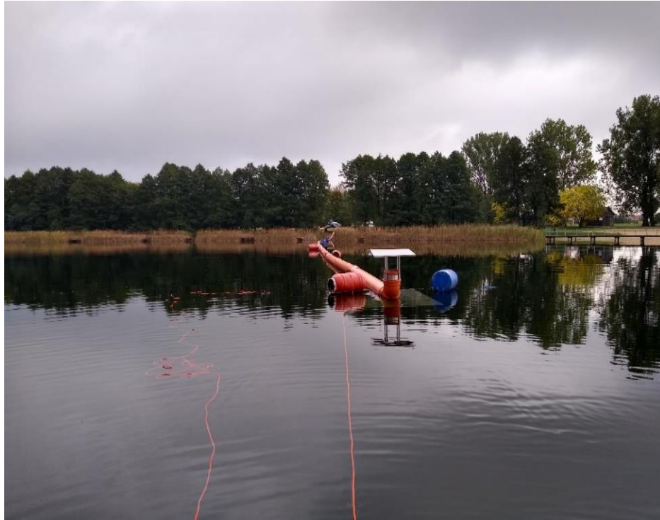
Photo 7. Deflector shield of the outflow pipeline inlet.
