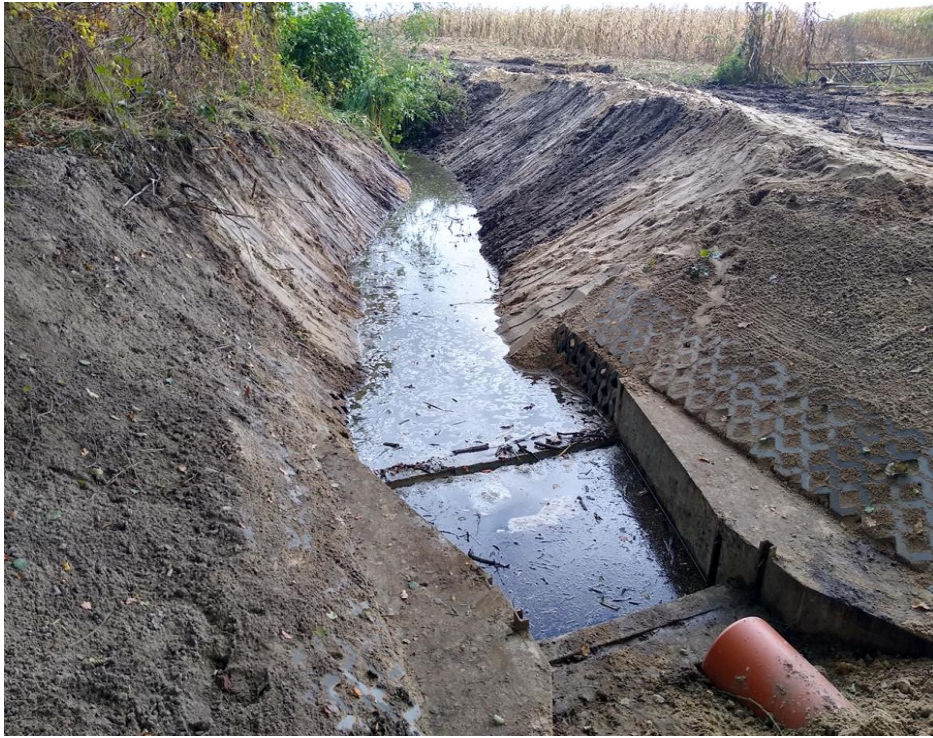
Photo 10. Construction of dam's inlet.
