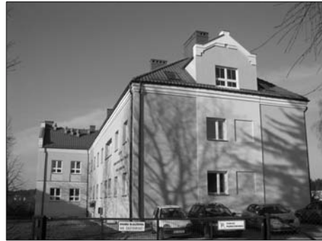
Fig. 2. The building of the Institute of Animal Reproduction and Food Studies, the Polish Academy of Sciences (PAN) in Olsztyn after the renovation and expansion. A view from the south-eastern angle. Photo: B. DEJA, 2008
