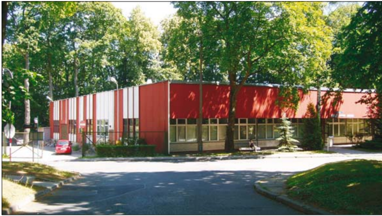
Fig. 8. A one-storey pavilion at 4 Heweliusza Street, photo: M. ZAGROBA
